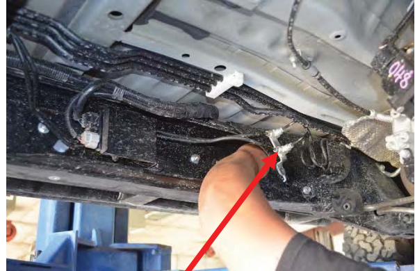
Bracket and lines moved in order to allow installers arm to fit into frame cutout
